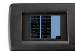
Chiller status display
